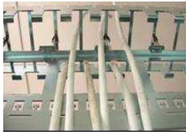
Pass two cables per cut-out, one of them through the panel square holes for the connector on the lower side
