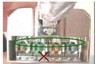
Check there are no cut-wire fragments left and re-check the correct position of the foils
