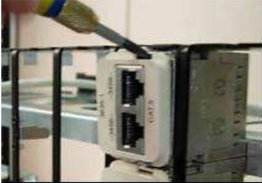
If necessary AMP CO Plus Inserts may be easily removed using a flat screwdriver (having previously removed the faceplate)
