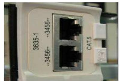
Additional identification of the ports may be achieved by using Icons, Labels for Dual Inserts and labels on the flat surfaces of faceplates
